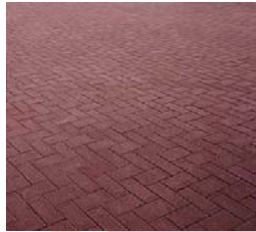
Concrete Pavers Donated by Alley-Cassetty
